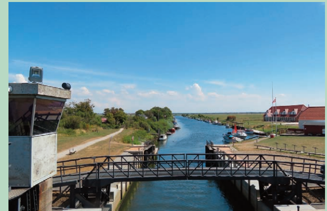
During storm surge, Kammerslusen is closed, thereby keeping the inhabitants of the marshlands safe from flooding. Photo: Charlotte Lindhardt.
